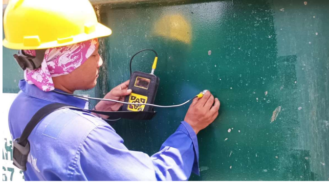
Figure 4. An ultrasonic thickness gauge is used in the inspection process
