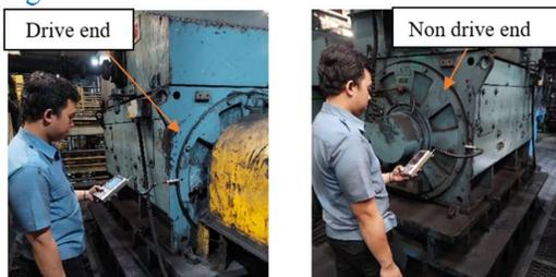
Figure 1. Measurements at the drive end and non-drive end positions
