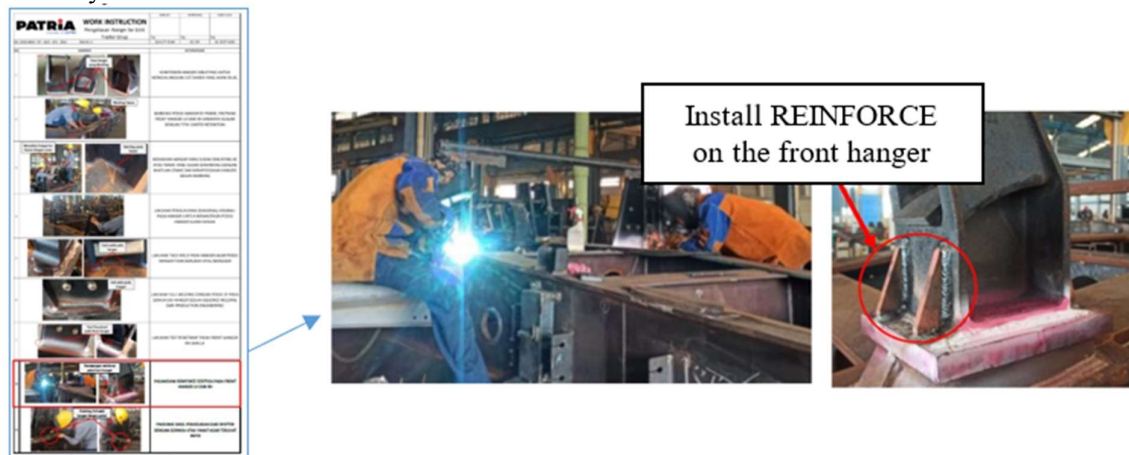
Figure 5. Hanger welding work instructions
